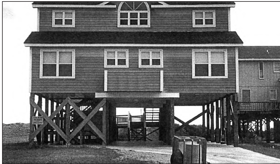
Figure 10-10. Diagonal bracing using dimensional lumber
